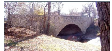
Phalen Park Stone Arch Bridge
